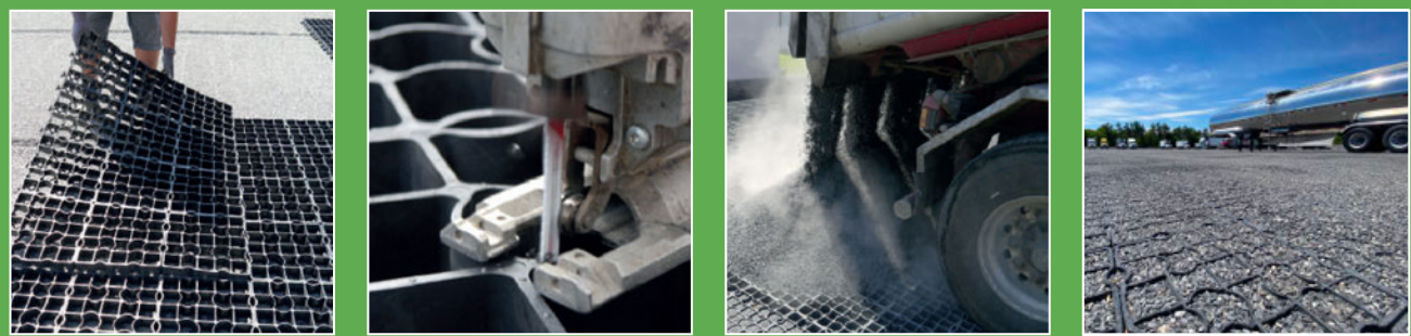
STEP 1. LAY STEP 2. CUT STEP 3. FILL STEP 4. IT'S DONE!
